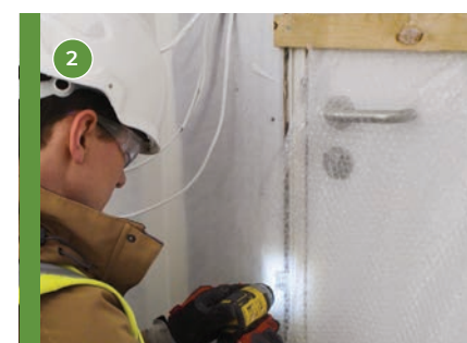
2 Level the doorset using the fixing brackets.
