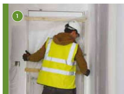
1 Position the doorset within the structural opening.
