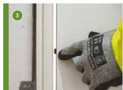
3 Use the Quick2Gap pads to ensure a 3-4mm gap between the door and frame.
