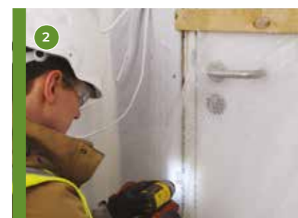
2 Level the doorset using the fixing brackets.
