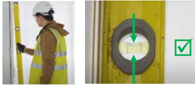
Once all the fixing brackets are secured, double check the Doorset is level in each plane and the 3mm gap has been maintained. Adjust if required.
