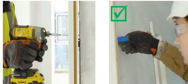
Insert solid packers between the frame and the wall at the fixing points. Note; the packers should be the same width as the frame section less allowance for appropriate fire stopping. This will avoid the frame distorting.
