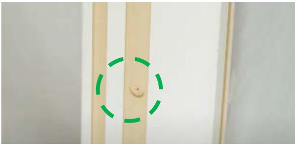
From the push side, the Joiner can quickly locate the frame's primary fixing points, which are pre-machined within the door stop channel.
