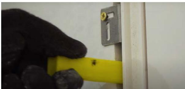
The Joiner using a wedge can easily adjust the gap between the door and frame to achieve a 3mm gap.
