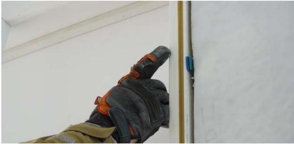
Machined into the edge of the frame is the groove for the adjustable architrave.
