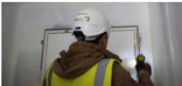
Adjust the position of the Doorset to ensure the hinge jamb is level in each plane and then tighten the fixing brackets along the hinge side jamb, packing underneath the brackets if required.
