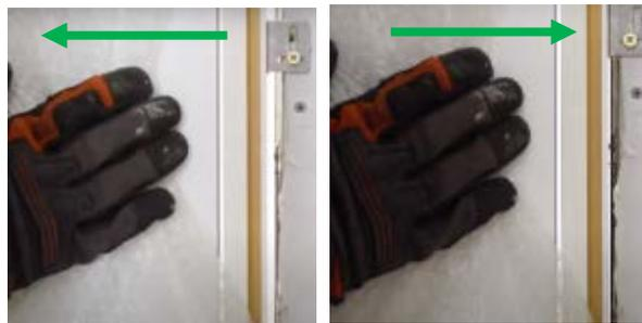
The 8nr adjustable fixing brackets allow the Joiner to alter the fitting position of the Doorset to take into account uneven finishes and sizing issues within 5mm
