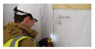
Before the transit braces are removed, the Joiner should <u>loosely</u> secure the Doorset into the opening.
