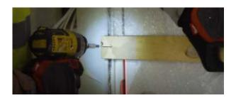
Once loosely secured into the opening, the transit braces and bubble wrap can be removed.
