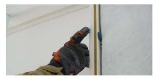
Machined into the edge of the frame is the groove for the adjustable architrave.
