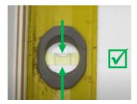
Once all the fixing brackets are secured, double check the Doorset is level in each plane and the 3mm gap has been maintained.
