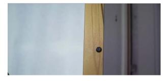
Having achieved the correct 3mm gap between the door and frame, the Quick2Fit pads can now be removed.
