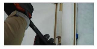
To secure the frames during transit and installation, the Doorsets are fitted with removable transit stops
