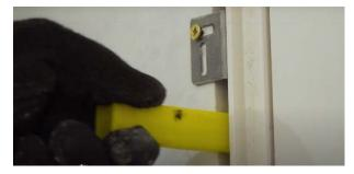
The Joiner using a wedge can easily adjust the gap between the door and frame to achieve a 3mm gap.
