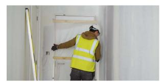
The Doorset should comfortably fit flush into the structural opening.
