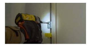
Once the Quick2Fit pads are touching the frame, the fixing brackets on the latch jamb can be secured, whilst ensuring the Doorset is level in each plane and the 3mm gap is maintained. Pack underneath the brackets if required.
