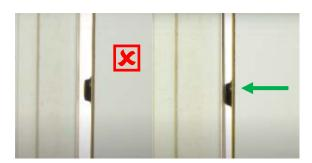
To retain fire, smoke and acoustic certification, as well as providing for future movement install to a 3mm gap.
