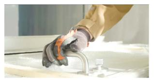
Doorsets are palletised "head to toe" so that pre-fitted ironmongery is not damaged during transit.
