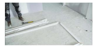
Architraves are provided loose, pre-sized, mitred and machined for Hoffman fittings, for the rapid installation without further cutting.
