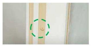
From the push side, the Joiner can quickly locate the frame's primary fixing points, which are pre-machined within the door stop channel.
