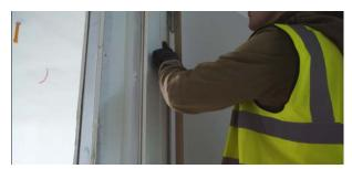
Once removed, the pre-cut door stops can be quickly fitted into the stop channel within the frame. The joiner can then fix the door stops in place, hiding the frame fixings.
