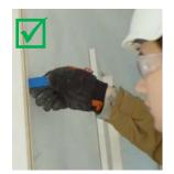
Insert solid packers between the frame and the wall at the fixing points. Note; the packers should be the same width as the frame section less allowance for appropriate fire stopping. This will avoid the frame distorting.
