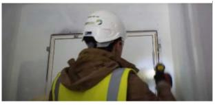
Adjust the position of the Doorset to ensure the hinge jamb is level in each plane and then tighten the fixing brackets along the hinge side jamb, packing underneath the brackets if required.
