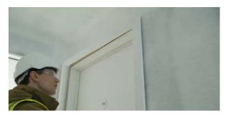
Once assembled the architrave set can be fitted into the architrave groove in the frame and pinned in place along the iambs.
