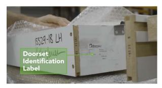
Each Doorset is clearly labelled so that the Joiner can quickly identify its correct location.
